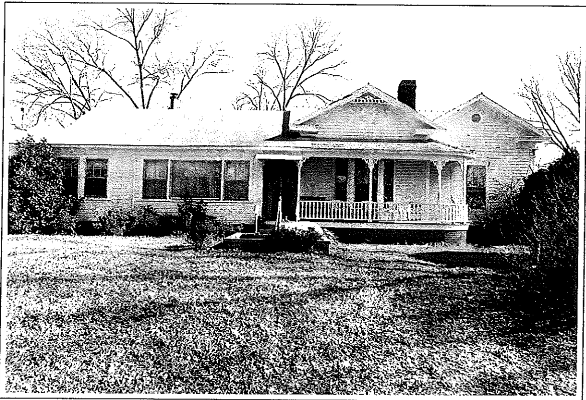
Dr. W. N. Tate Farm (#G). West elevation of farmhouse (post-1910 additions to left of porch).
