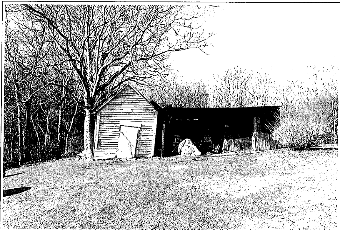
House (#K). Frame shed and lean-to shed.
