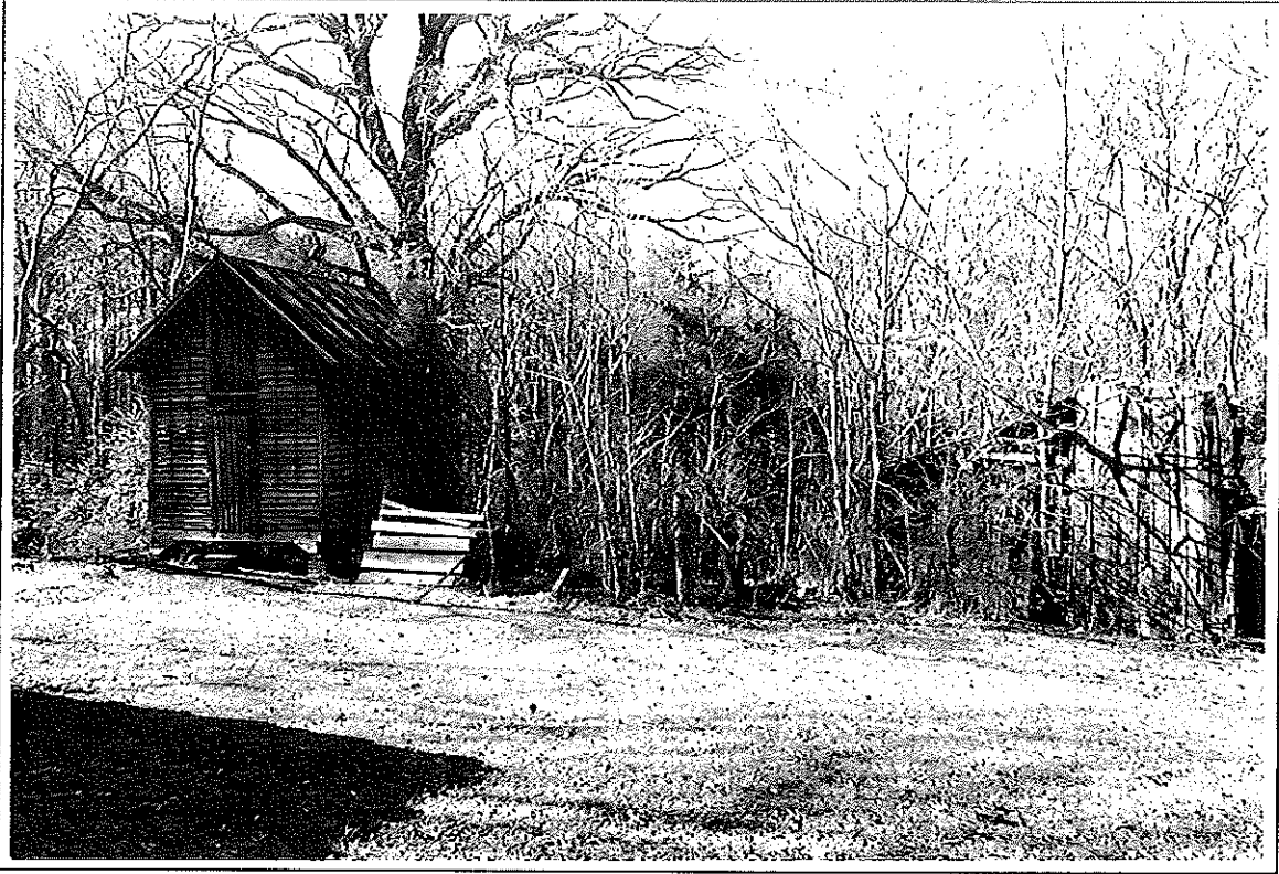
House (#K). Corn crib and collapsed barn.
